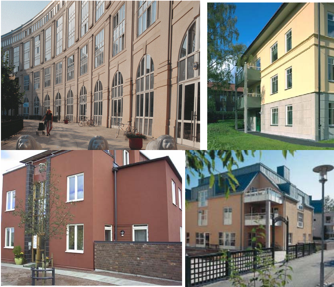
Figure 4.6 Examples of façade designs of modern Swedish precast concrete dwelling buildings. Top left: Concrete surface similar to sandstone obtained by washing of the fresh, coloured concrete. ‘The Arch of Bofill’. Stockholm, Top right: Painted elements with surface structure similar to rendering and joints used as design feature. Frösön, Jämtland: Bottom left and right ‘Joint free’ sandwich elements with lightweight aggregate in outer leaf. Stockholm. Also compare cover photo, showing a painted sandwich element façade.
