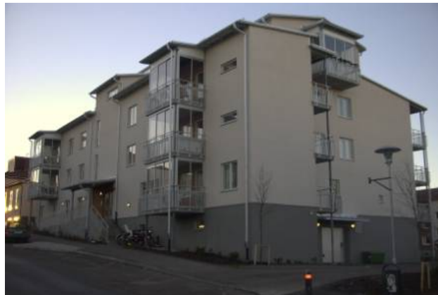
Figure 7.6 Example D. Façades facing to the East and North. Photo by the author.
