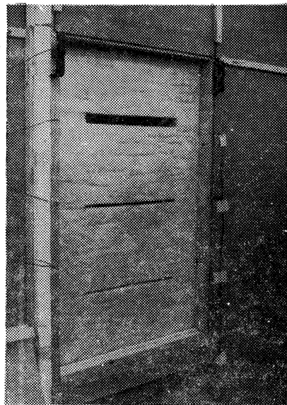
FIG. 6.15-6.16. Vertical and horizontal slits in the insulation. Viewed from cold side before the erection of the covering board.
