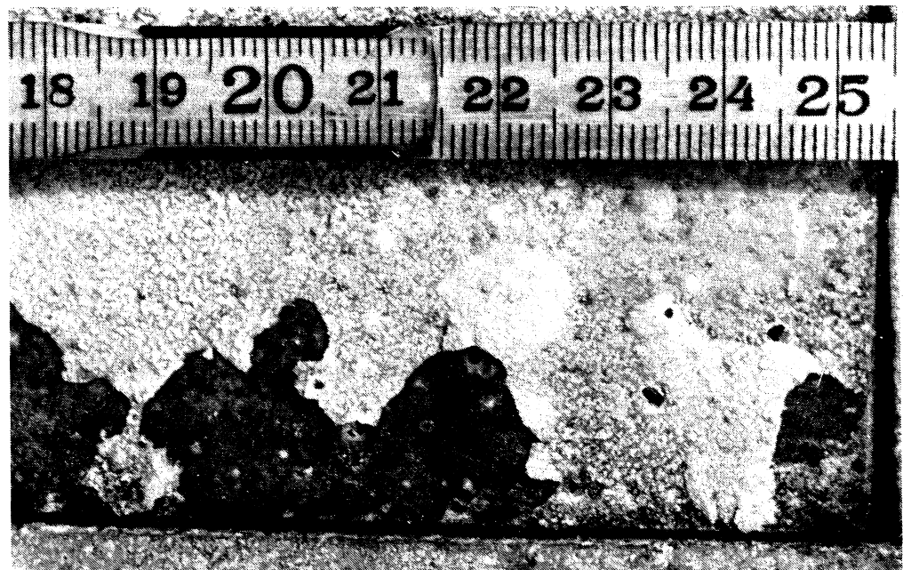
Figure 9.6 : Detail of 0,60 mortar prism with partially lost layer of magnesium hydroxide.
