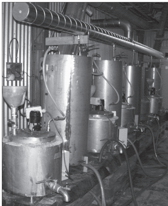
Figure 2. The systems for pilot-scale continuous anaerobic digestion.
