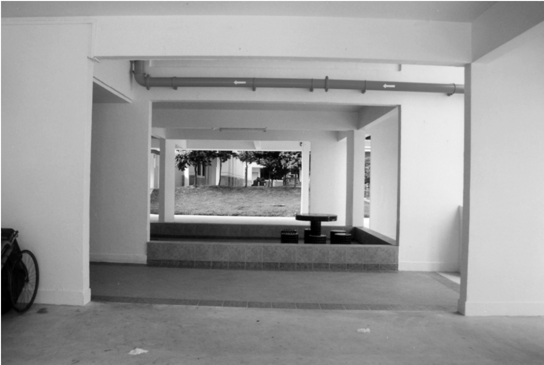
The void deck under an apartment block.
