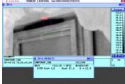
Figure 10: Ventilation intake over the kitchen window.
