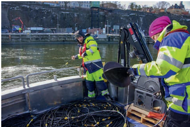
Figure 4 Deployment of electrode cable in progress.
