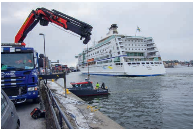
Figure 5 Measurement in progress with the ferry passing over the survey line. The survey boat used for deployment of the electrode cable, sonar depth mapping, etc., is visible in the foreground. The truck was used to place a concrete block on the sea bottom, which was used as anchor to secure that the start position of electrode on cable was fixed when deploying it.
