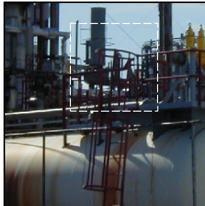
Fig. 6. (1.6 MB) Movie of ethene leakage. By sweeping the camera system over the polyethylene plant, a leakage was found. A visible image and a sequence of gas images are shown. The gas-correlated images are merged with the zoomed visible image. The ethene gas leakage was taken care of immediately by the operating personnel ( 3.8 MB version ).
