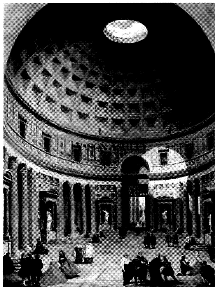
Figure 1 Pantheon, with its wide concrete dome, is an impressive structure from the ancient Roman Empire. The building was erected about 2000 years ago.
