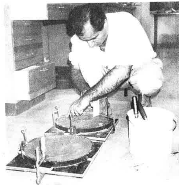
Fig. 7. Protective layer of mortar reinforced with chicken wire.
