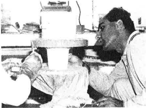
Fig. 8. Application of epoxy resin at the edge of the specimen.
