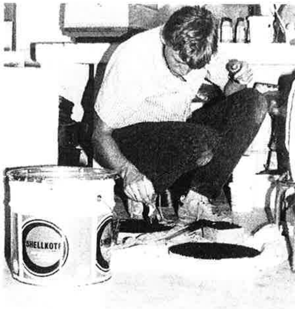
Fig. 6. Painting the bituminous emulsion in proposal 3.
