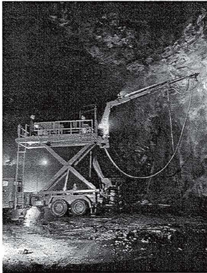
FIG 9. Robotized spraying of fibre shotcrete. (Photo: BESAB)
