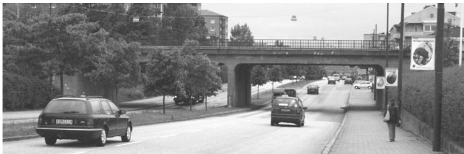
Figure 7.1 Photograph of the investigated bridge.
