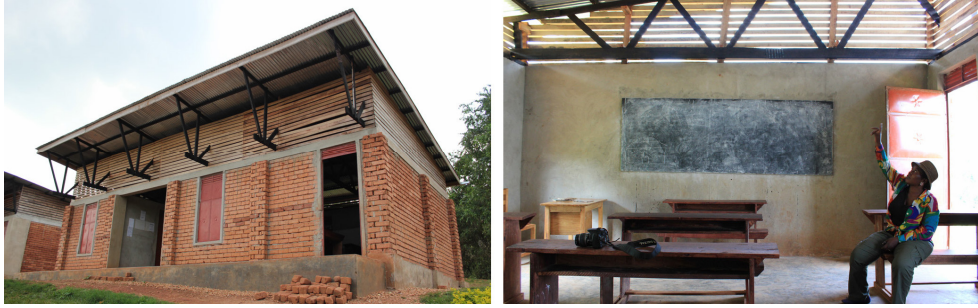
Figure 18: Picture of a classroom building in the elementary school
