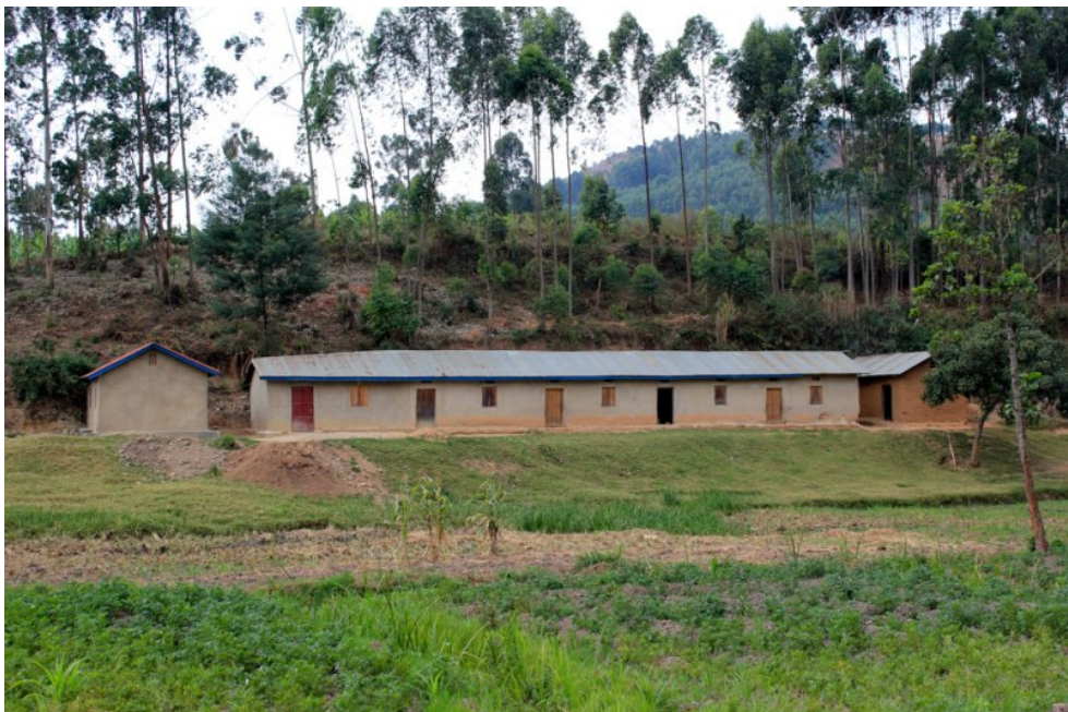
Figure 5: Photo illustrating the three main buildings on site From left to right: Office building, school building and storage/kitchen building
