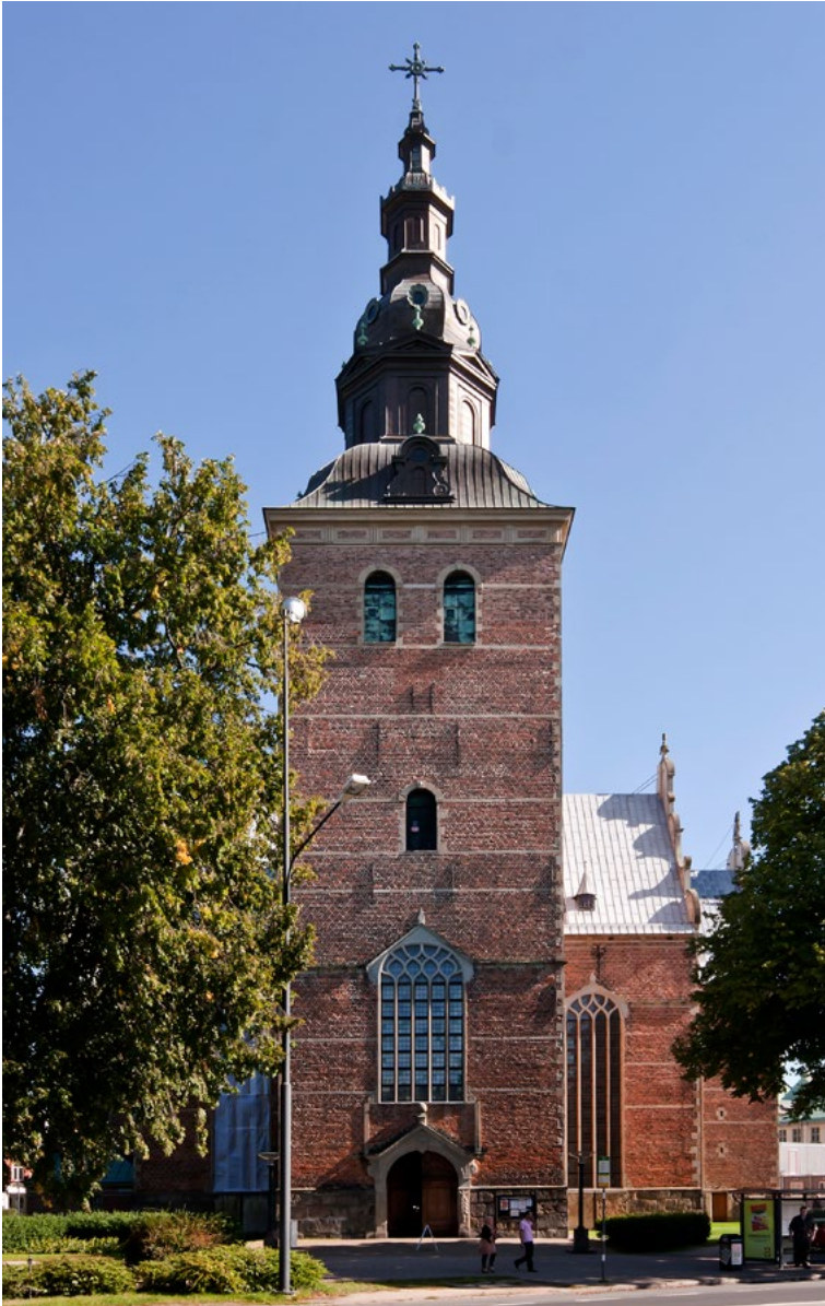
Figure 50 Exterior of the Trinity Church in Kristianstad, built 1618-1628. The architects were Lorenz van Steenwinckel and Hans van Steenwinckel the Younger. Photo: David Castor, CCO i.o., Wikimedia Commons.
