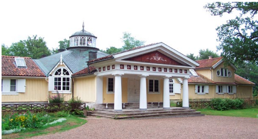
Figure 97 Fredric Henric af Chapman and Carl August Ehrensvärd, Skärva, 1787. The panelling covering the timbered construction is of later date. Photo: Henrik Sendelbach, CC BY-SA 3.0, Wikimedia Commons.
