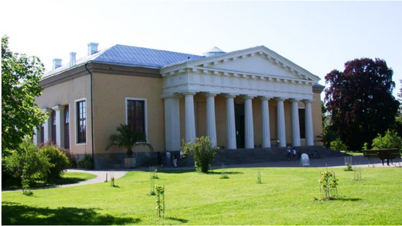
Figure 110 The Linnaeanum, main building in the Botanical garden in Uppsala, inaugurated in 1807. East façade with Doric portico. Photo: Riggwelter, Public Domain, Wikimedia Commons.
