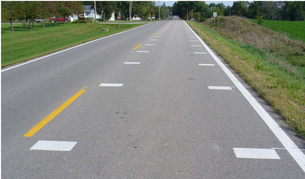
Figure 16. Transverse pavement marking bars (Fitzsimmons et al., 2009).
