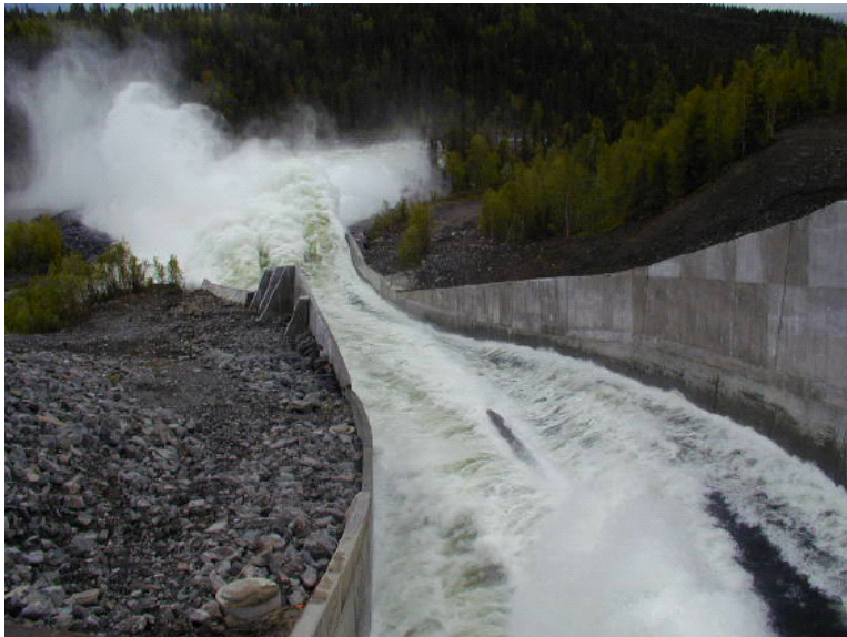
Figure 6-6 – Discharge of water.
