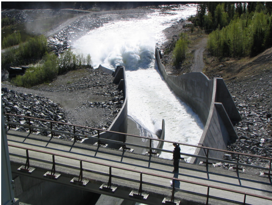
Figure 6-1 - Ajaure spillway chute during discharge test.
