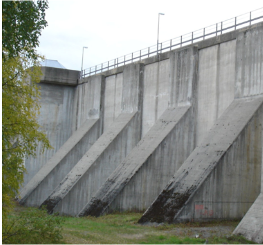
Figure 2-2 - Buttress dam at Stornorrfors.
