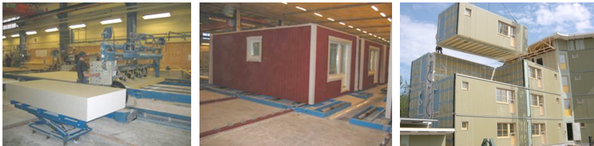
FIG 2: Modular house production
