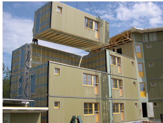
Figure 3. Modular house production.
