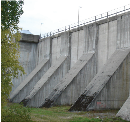
Figure 4-2 - Buttress dam at Stornorrfors.
