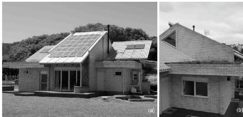
Figure 3.21: Experimental building with the green, ceramic and metal roofs: North façade view (a) and exterior view of bedroom 2 (b) (Source: Parizotto and Lamberts, 2011).
