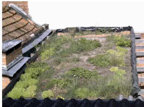
Figure 3.4: Lack of plant coverage in a green roof built in Porto Alegre (Krebs, 2005)
