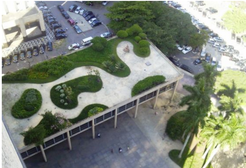
Figure 3.10: Intensive green roof at Gustavo Capanema Palace, in Rio de Janeiro (Fracalossi, 2013)
