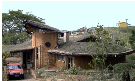
Figure 3.3: Complex self-constructed green roof (Krebs, 2005)
