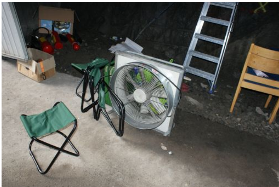
Figure 11. The mobile fan that was used to distribute smoke and acetic acid in the tunnel.
