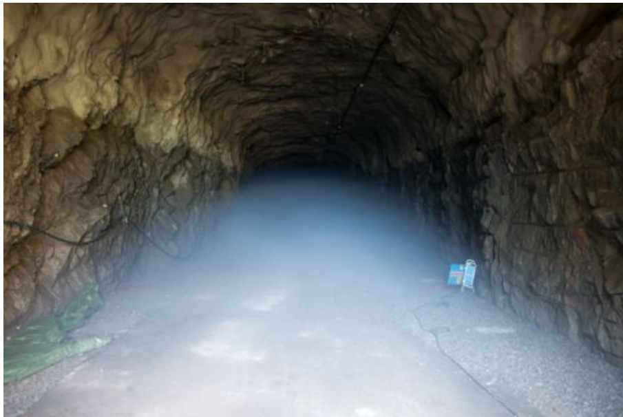
Figure 1. The geometry of the tunnel and the tunnel wall covering. The smoke discernible in the picture had been added artificially. Photo: Stefan Svensson.
