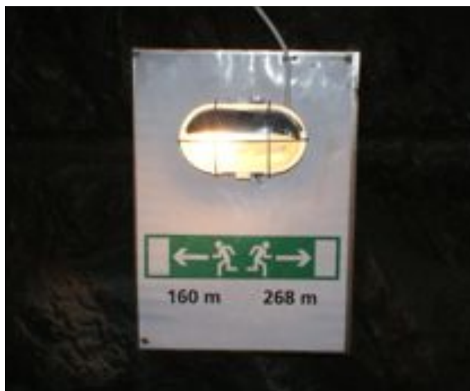
Figure 5. One of the emergency signs used in the experiment, more specifically the first sign on the right side of the wall.
