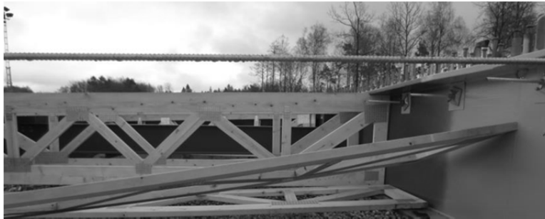
Figure 6.17 A timber-frame falseworks used in a bridge application.
