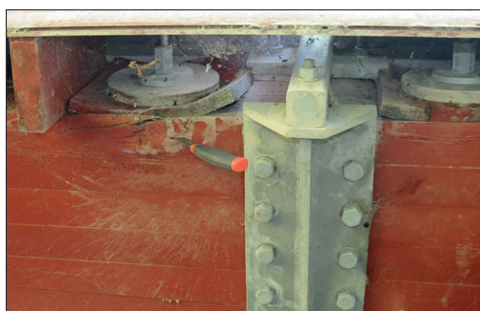
Figure 2.2: Damaged cross-laminated timber bridge. Photograph courtesy of A. Pousette & P.A. Fjellström.
