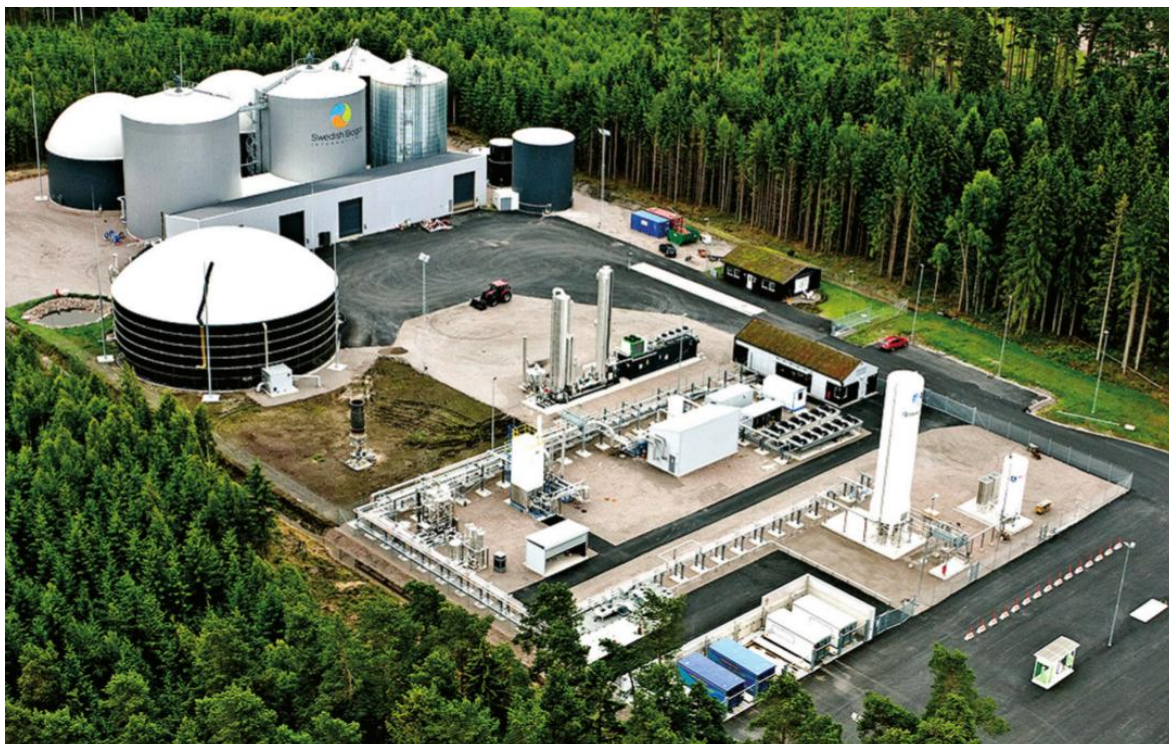
Figure 37 The Lidköping Biogas plant. In front the filling station is shown, and behind that the liquefaction unit is situated.
