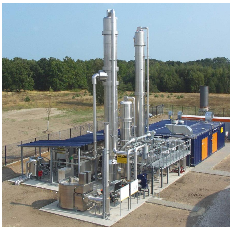
Figure 27 An organic physical scrubber with a capacity of 1100 Nm 3 /h of raw biogas. Image from Haase Energietechnik.
