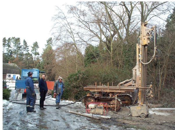
Fig. 2: Drilling a borehole to a single family dwelling
