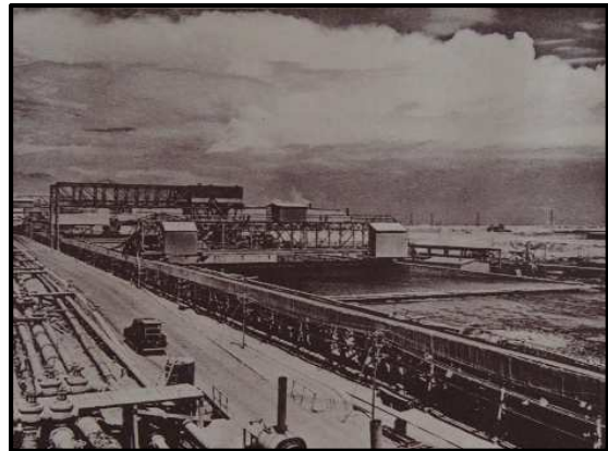
Leaching tanks at Chuquicamata
