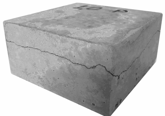
Figure 6. The crack in the upper part of the specimens of w/c-ratio 1.0 appeared at the level of the top paper layer.
