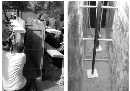
Figure 6 & 7. Left: ramming the first layer. Right: installing the formwork. Photo credit: M. Dabaieh.
