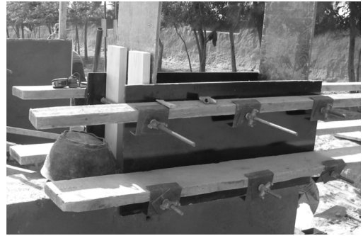
Figure 5. The formwork when assembled to ram a new layer. Photo credit: M. Dabaieh.
