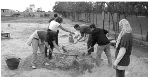
Figure 4. Participants mixing & preparing the soil for ramming Photo credit: M. Dabaieh.
