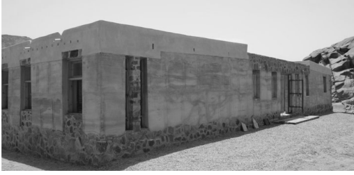
Figure 1. Center for building crafts in Sinai built with rammed earth and stone. Photo credit Nashwa Ibrahim.
