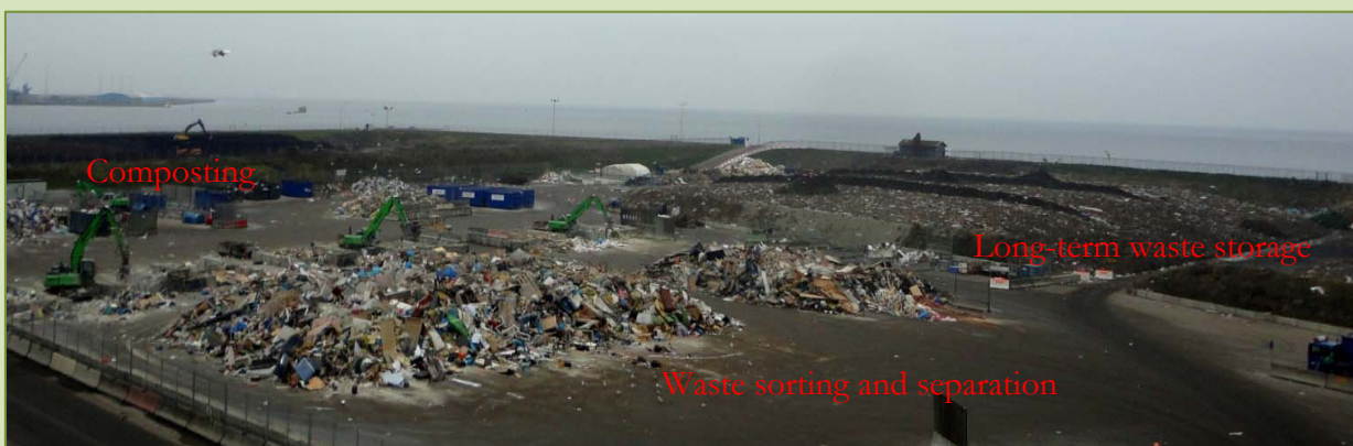
SYSAV Waste Sorting, Treatment and Storage Site in Malmö, Sweden
