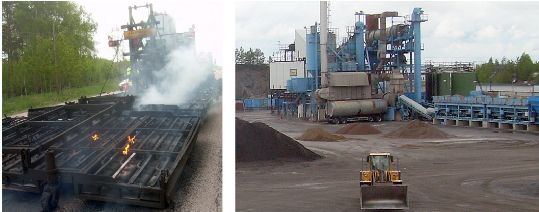
Figure 7. Recycling of asphalt on site and at an asphalt plant.
