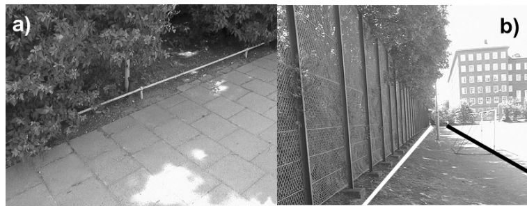
Figure 11 Example of resistivity profiling close to an iron fence. a) This fence is placed 1 m outside the fence in b) and consists of a small iron rail that is in very good galvanic contact with the ground. b) A fence isolated from the ground by concrete foundations and the position of two resistivity sections.
