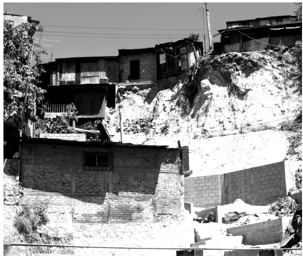
fig 8: Location of a slum community on marginal land and steep slopes
