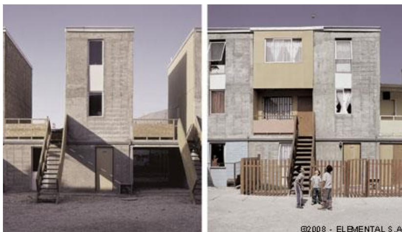
Figure 12: Project at Iquique, Chile showing to the left the delivered houses and at the right its expanding possibilities
