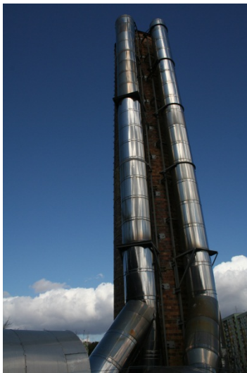
Present and past meet – chimney for one of the gas-power boiler plant operated by OPEC mounted on the old.
