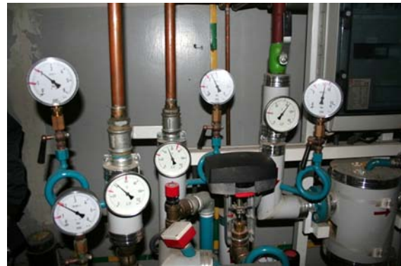
Gauges on a heat exchanger connect to a small gas boiler operated by OPEC.
