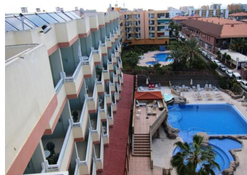
Las Walkirias rooftop is utilised for solar thermal panels to heat the pool below.
