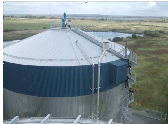
Biogas plant in Sweden
