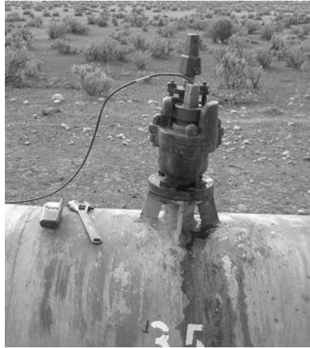
Figure A.12: Pressure transducer mounted on the fire hydrant plug
