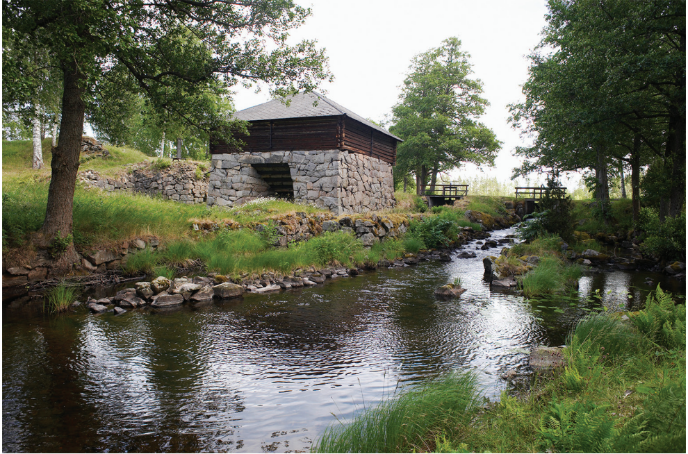
Fig. 58. Ruin of a blast furnace from the eighteenth century by the factory of Silvhytteå in the municipality of Hedemora, province of Dalarna (photo: Bengt A. Lundberg, Swedish National Heritage Board)
