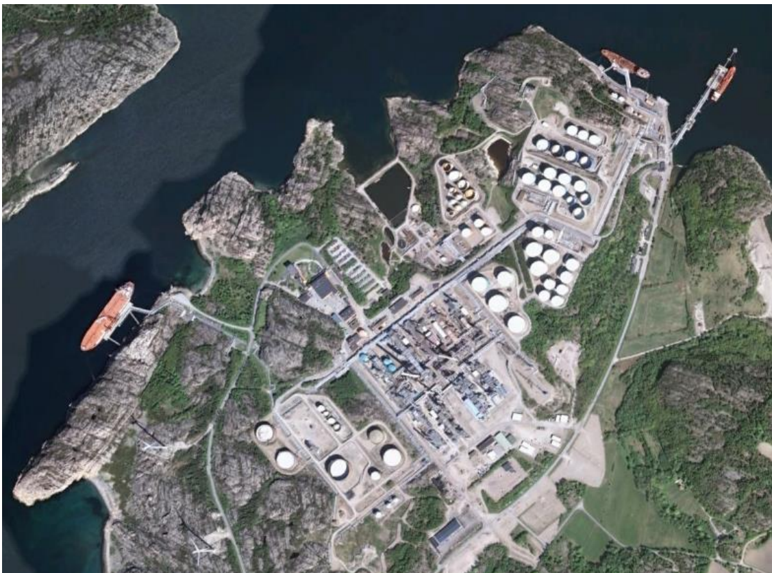
Figure 9 Satellite image of Preemraff Lysekil situated by Brofjorden on the Swedish west coast. On the left hand side is the crude oil import harbour and in the upper right corner is the product export harbour. Image from Google Earth (Lantmäteriet/Metria).
