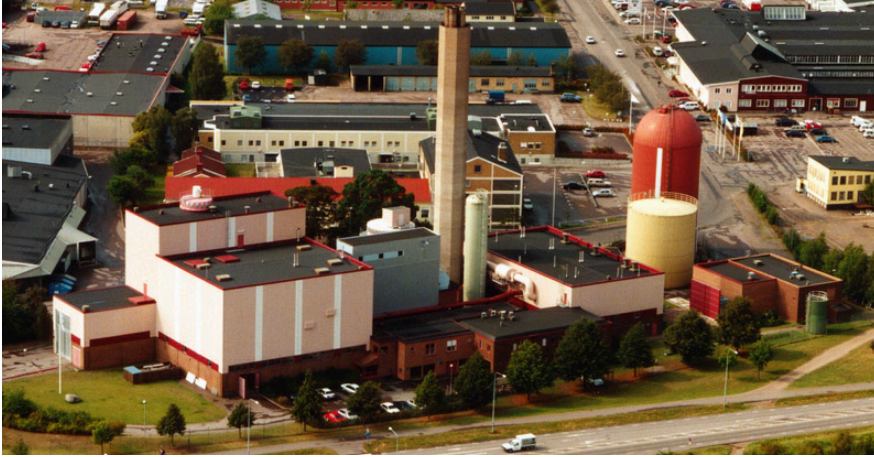
Figure 1.2: An aerial view of the central heating plant "Draken" of Kalmar.
