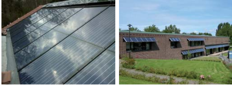
Figure 1.6 Left, building-integrated PV modules. Right, PV modules working as a sunshade. Photo: GAIA Solar.
