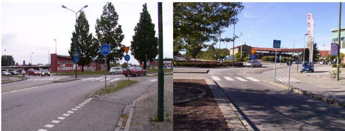
FIGURE 17 Roundabouts with different location of the yielding sign and line, Sallerupsvägen/Scheelegatan and Köpenhamnsvägen/Erikslustvägen, Malmö City
