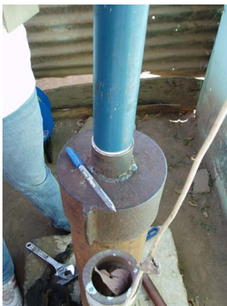
Fig. 6 Airtight coupling using a casing cap with a fitting for the slug test equipment in the centre. Pen for scale.
