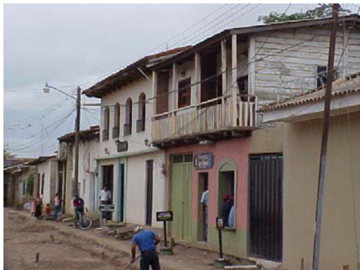
Partial view of the existing structures
