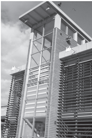
Figure 3: Illustration of integration of the Solar Window into the glazed façade of a staircase of an ecological exhibition building in Malmo.
