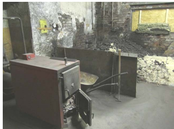
A “dirty” boiler and accompanying coal supply.
