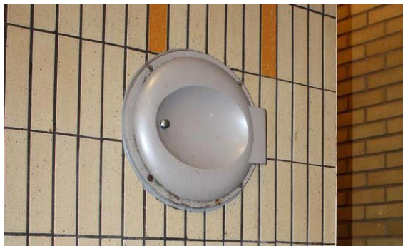
A locked waste chute in Sweden
