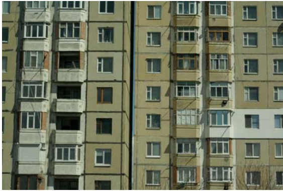
Residential building block in Chișinău, Moldova
