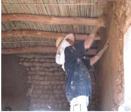
Figure 5.30 Plastering layer is thrown on the walls.
