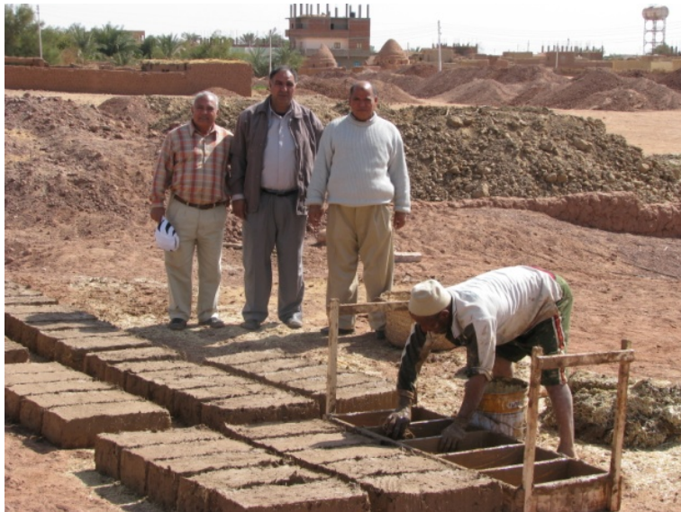
Figure 5.12 Mud brick casting using the first alternative of the mould and the representatives from the local municipality visiting the site to follow the work in process.
