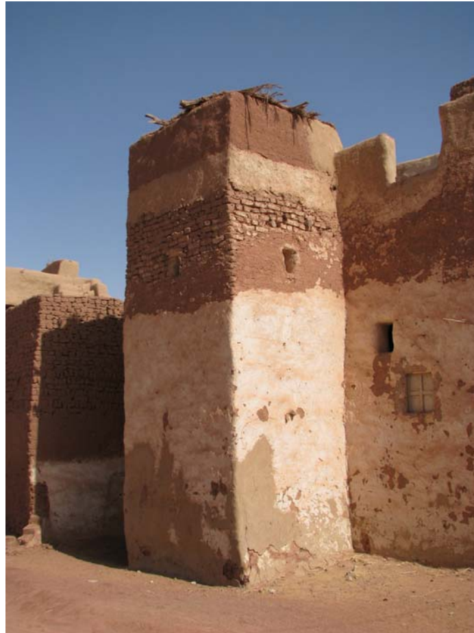
Figure 4.53 Dry toilet (compost) with roof covering from palm ribs and leaves for shade. The toilet has an opening in the bottom of this tower to collect the wastes when they are completely dry twice a year. The wastes are used as soil fertilizers or fuel for ovens.
