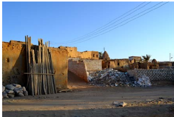
Figure 1.2 Deterioration of vernacular architecture and replacement of vernacular houses with concrete skeleton and white brick ones in the Baharia oasis.
