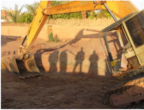
Figure 5.15 The site while digging.
