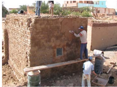
Figure 5.33 Exterior wall rendering using plastering trowels.
