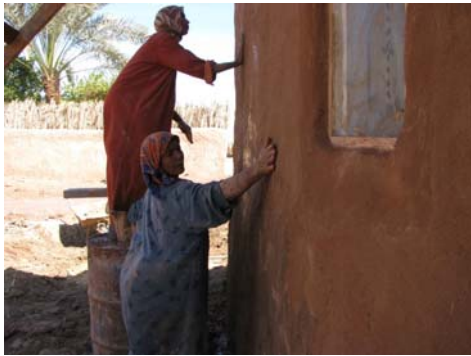
Figure 5.32 Exterior wall rendering with the help of Balat ladies using traditional manual techniques.
