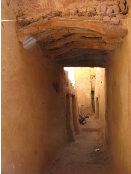
Figure 2.5 Example of shaded tunnelled alleys.
