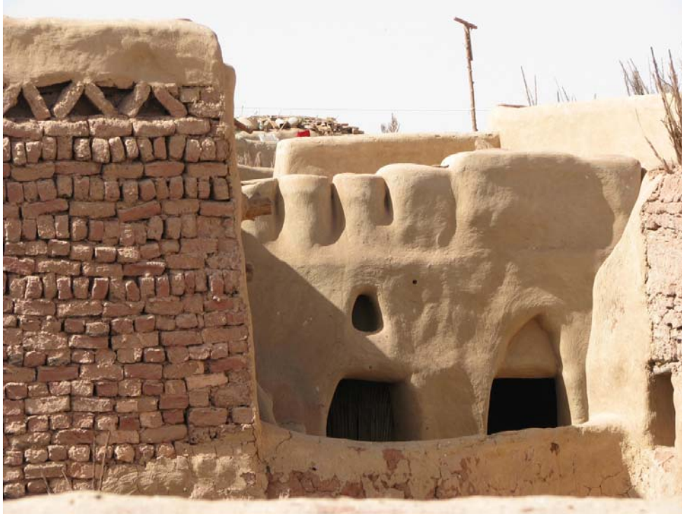
Figure 4.28 Parapets, openings and wheat storage are pieces of hand sculptures in Balat.
