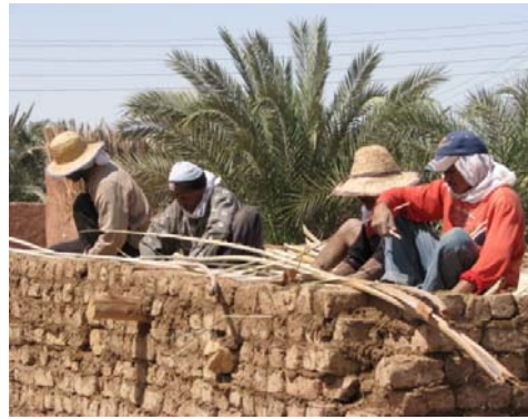
Figure 5.28 Placing palm leaves on top of reeds.
