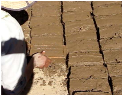
Figure 2.18 Process of casting mud brick in the Dakhla oasis.
