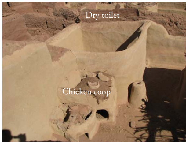
Figure 4.46 Examples of the functions of a roof floor. Dry toilet with no roof covering and small chicken coop.
