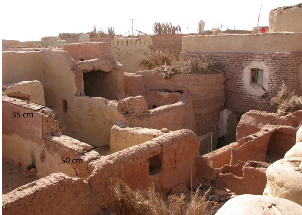
Figure 4.16 Cluster of houses in Balat showing the wall thickness of a second floor and a roof floor.
