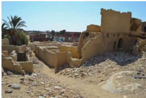
Figure 1.5 Deterioration of vernacular houses and replacement with concrete skeleton ones in the Farafrah oasis.
