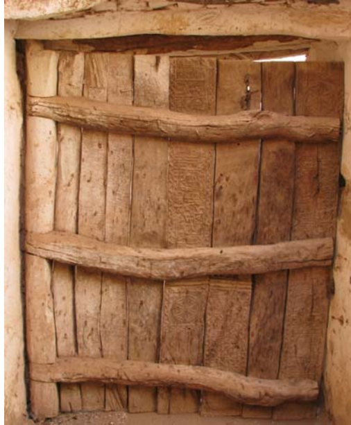
Figure 4.63 Mayor's courthouse entrance door showing special door design and craftsmanship in using local materials. Photo taken during site survey in 2009.
