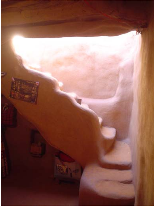
Figure 4.13 Staircase shaft function as wind catchers.
