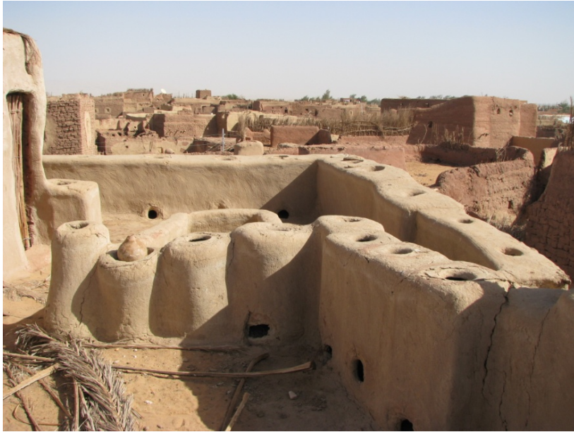
Figure 4.47 Mud pots for storage of grain on the roof floor.
