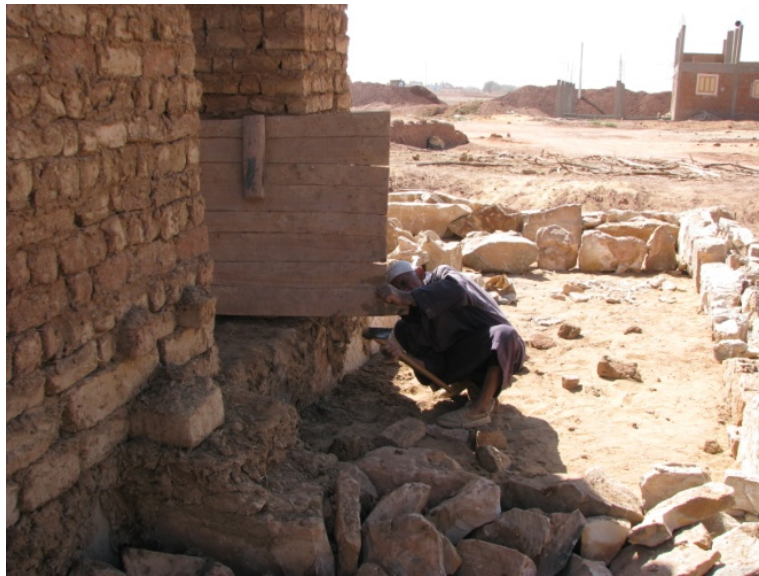
Figure 5.38 A senior local carpenter fixing the traditional door made from local wood.
