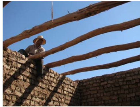
Figure 5.26 Placing the wood logs on the walls.
