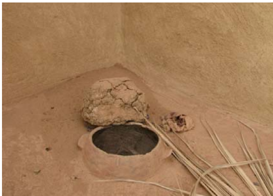
Figure 4.12 Bottomless pottery vessels serve both as skylights and ventilation openings.
