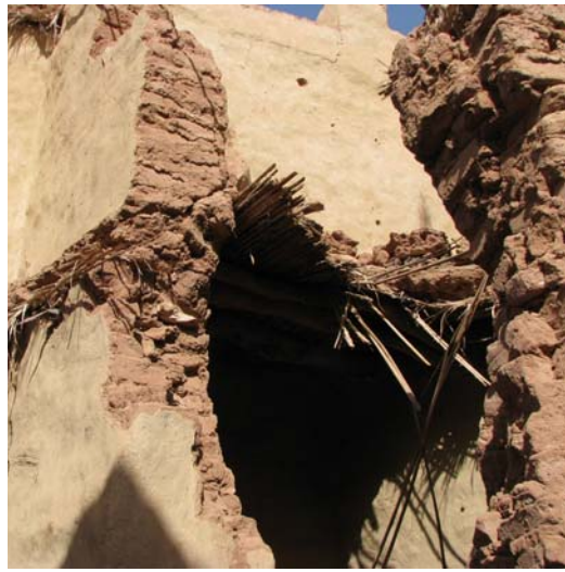
Figure 4.90 A part of a deteriorated house showing wall thickness made from mud bricks.
