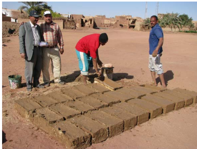
Figure 5.13 Mud brick casting using the second alternative of the mould. Youth were responsible for mud casting in shifts following seniors' instructions.
