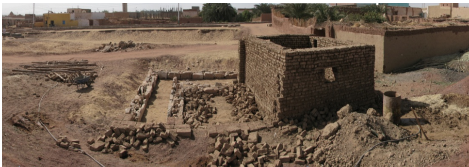
Figure 5.9 The site during construction for the neo-desert vernacular model, showing the foundation of the house and the room during construction.
