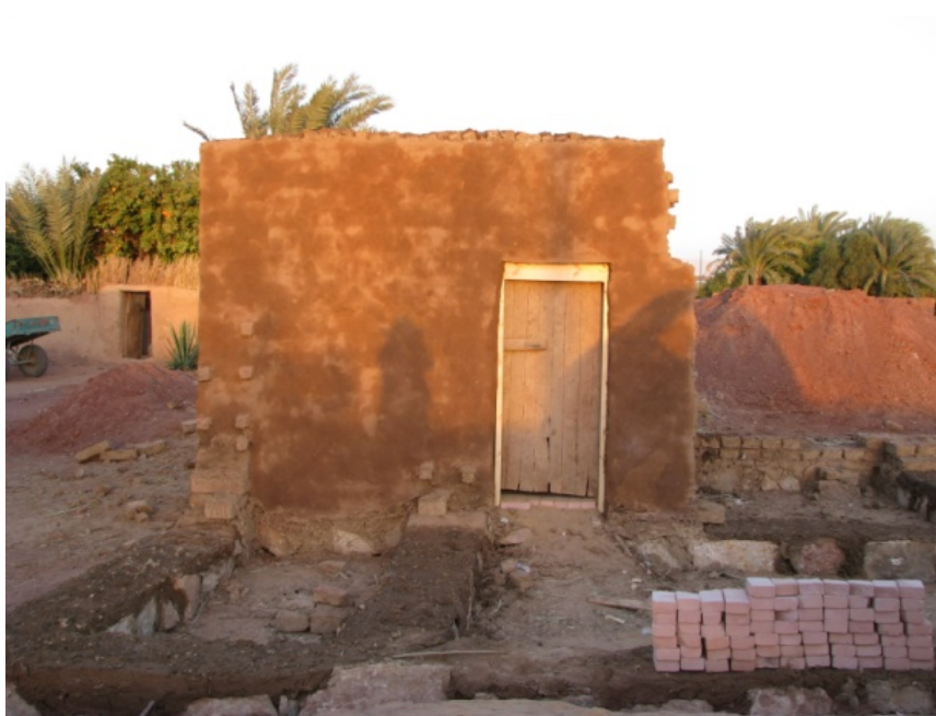
Figure 5.40 The finished room.
