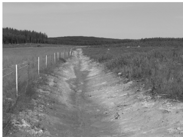
Figure 19. New Ditch on the Clearing, Farm CF 9
