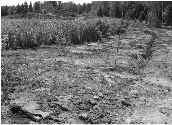
Figure 43. Piped Ditch Leading to the Clearing
