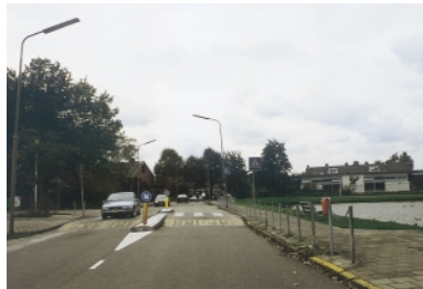
2. raised pedestrian crossing
