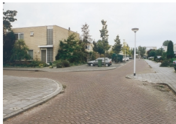
4. extended sidewalk at T-intersection
