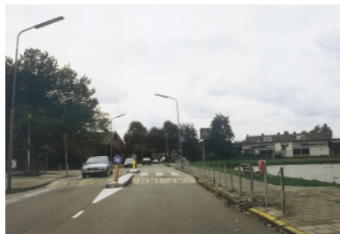
2. raised pedestrian crossing
