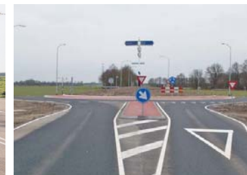
9. roundabout on extra-urban road
