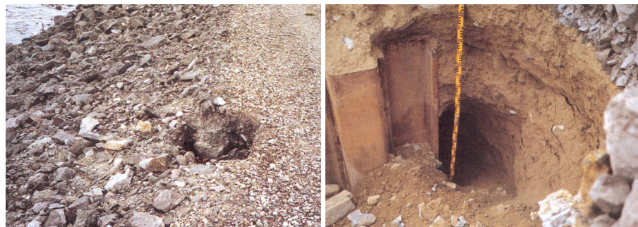
Figure 4. Two examples of effects from internal erosion in Swedish embankment dams. Left: Sinkhole, approximately 0.4 m in diameter, appearing on the upstream side of the crest. Right: Piping, approximately 1 m in diameter, through the dam core adjacent to a sheet pile. Foto: Gösta Johansson, AIB (WSP).
