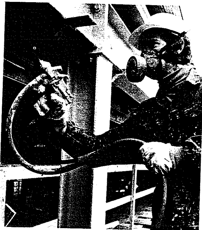
Fig. 11.1.4 a. Fire insulation of steel structure with fire retardant paints
