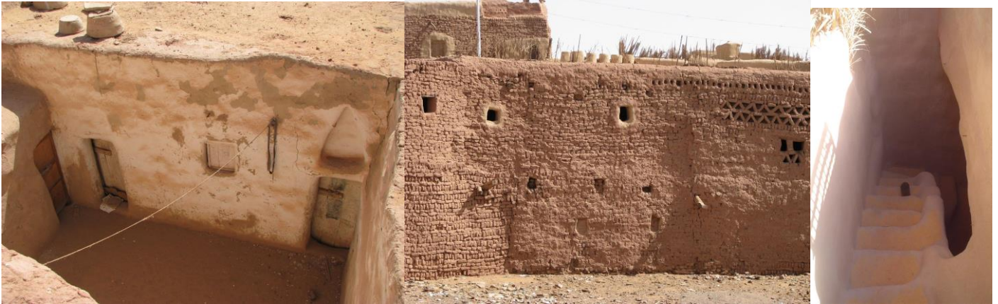
Figure 3: A collective shots for the Mayor house showing from left to right, the passive climatic responsive solutions in coping with hot climate like shaded courtyards, small windows facing prevailing favourable winds and staircase that acts as air shafts (Source: Dabaieh).
