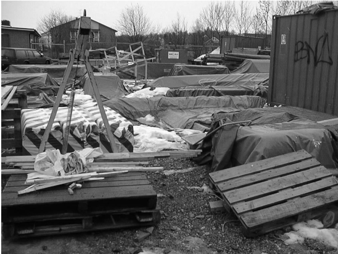
Figure 19: Construction materials on the site.
